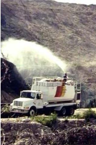
**HYDROGRASSING** has emerged as one of the most practical methods of establishing ground cover, particularly on slopes and difficult access areas. Because of the varied slurry capabilities, prepared ground surfaces can be covered in a single pass, thereby realizing a significant labor savings.
